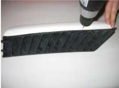
On the back of the scoop drill 2 holes for the rivets as shown on the picture. Leave at least 2.5mm (3/32" for the Imperial folk) space between the hole and the edge of the scoop.
